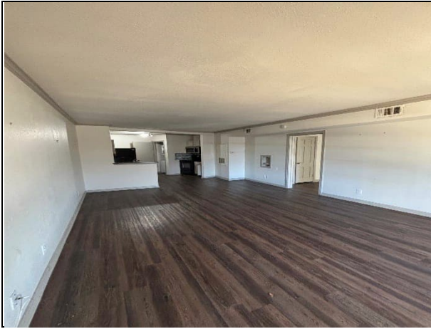
Photo #13 Asbestos containing finished drywall ceiling with texture (wavy).
