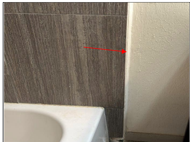
Photo #12 Asbestos containing finished drywall wall with texture (wavy).
