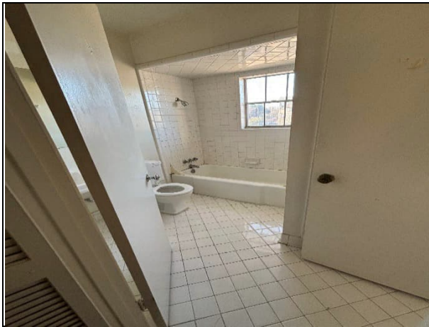
Photo #1 View of white ceramic floor tile with asbestos-containing thinset in Unit 17.
